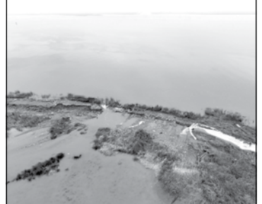
Van Sickle Island levee breach. Photo credit of California Department of Water Resources
