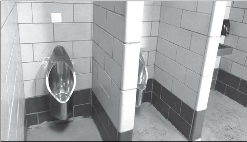
Restroom interiors at Rusch Park have been retrofitted by replacing all of the porcelain fixtures with stainless steel models at a renovation cost of more than $10,000.
