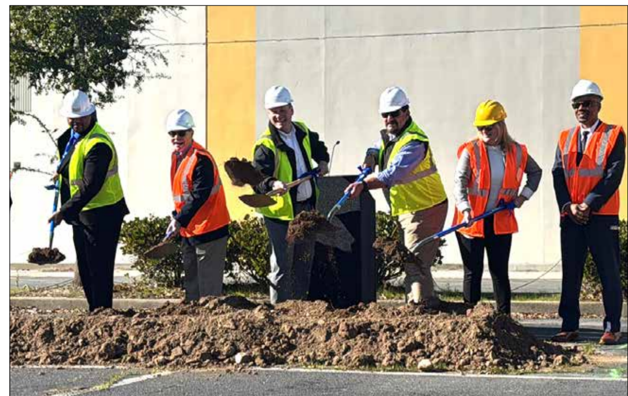
Ground has officially been broken to begin work on the Watt Safe Stay Community. Photo courtesy of Sacramento County
