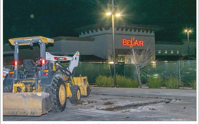
Construction is underway in the Bel Air parking lot to install a Tesla electric vehicle charging station, with completion expected in six to seven weeks. Photo by Gail Bullen
