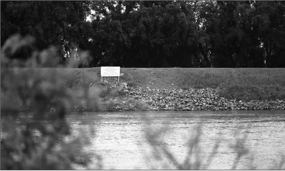
A repaired section of the levee near Isleton on the Sacramento River.
