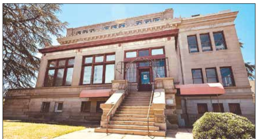
The historic Packard Library building at 301 4th St. in Marysville has stood for more than a century. Now largely vacant, the site is at the center of a legal effort by the city to reclaim ownership.
