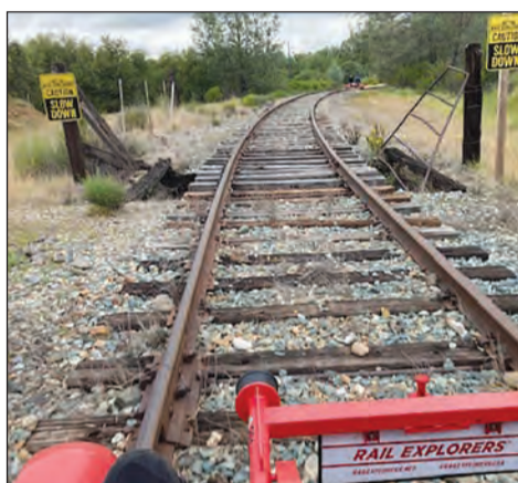
Signs on the downhill route warn of upcoming stops for grade crossings.
