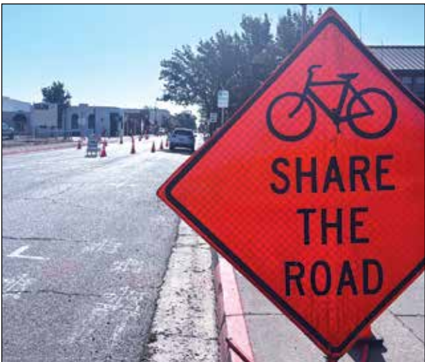
According to the City of Dixon’s website, construction is taking place from May 19 to June 27. Construction, conducted by Cal Water, starts at West A St. and stretches from First St. to Porter St. Photo by Kendall Brown
