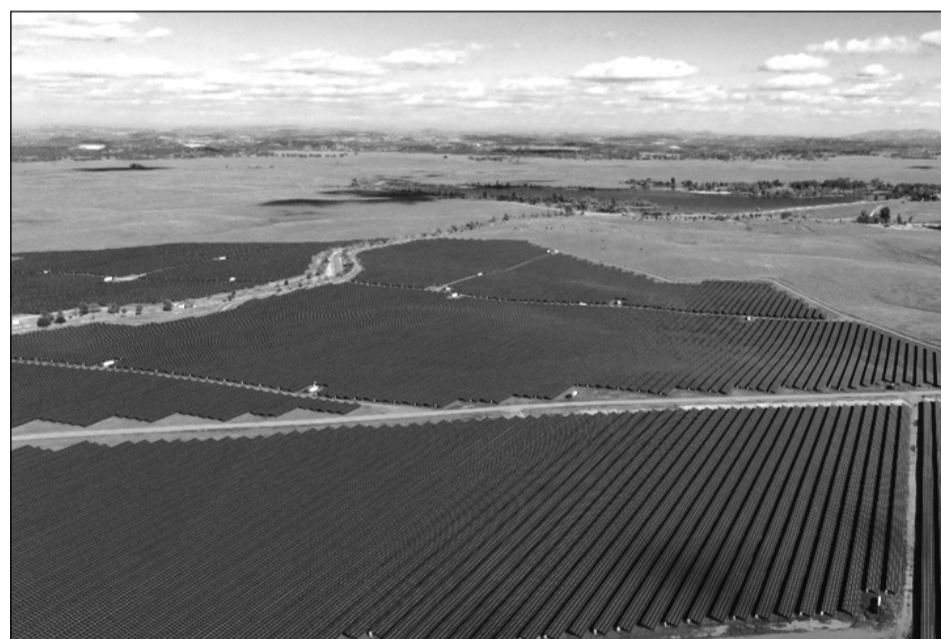
Rancho Seco's energy infrastructure includes a 160-megawatt solar facility, showcasing the Sacramento Municipal Utility District's commitment to clean energy generation. The innovative site combines solar power with sustainable land management through sheep grazing. Photo courtesy of Sacramento Municipal Utility District
