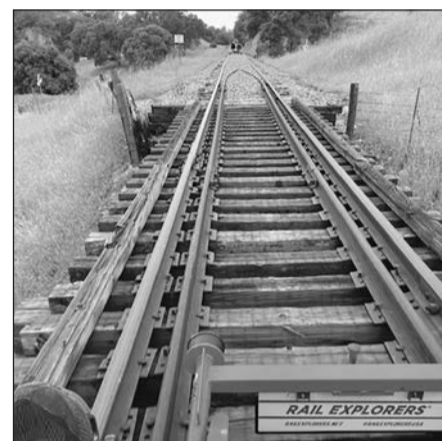
A railbike crosses the Highway 88 bridge.
