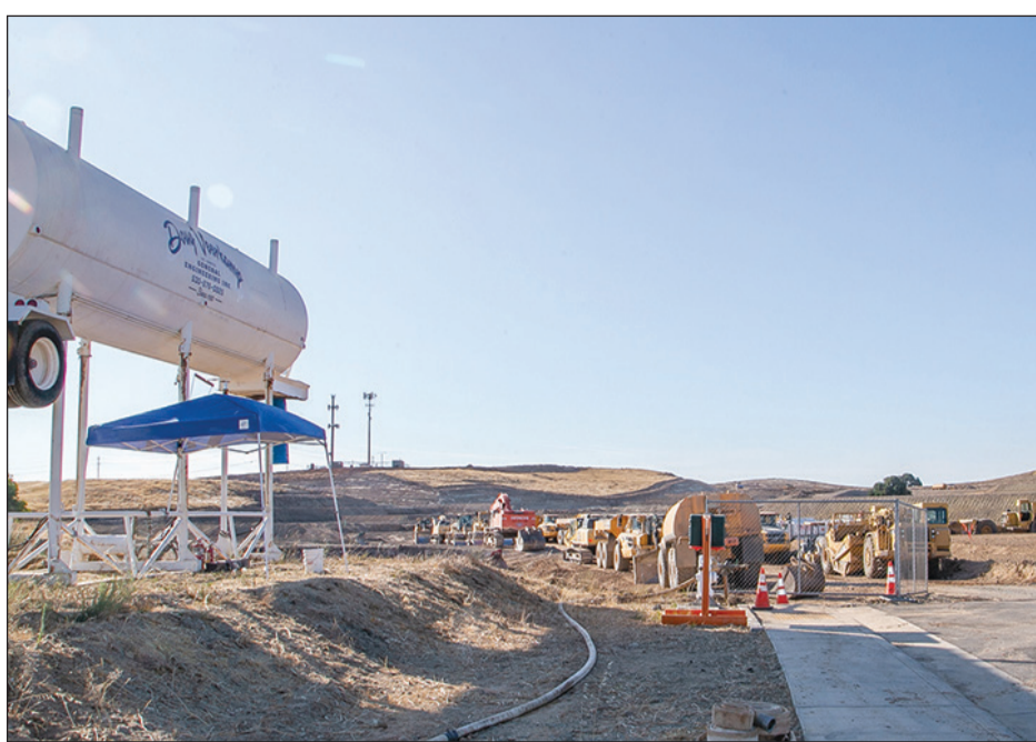
Veerkamp Engineering is currently grading Unit 2. Photo by Gail Bullen
