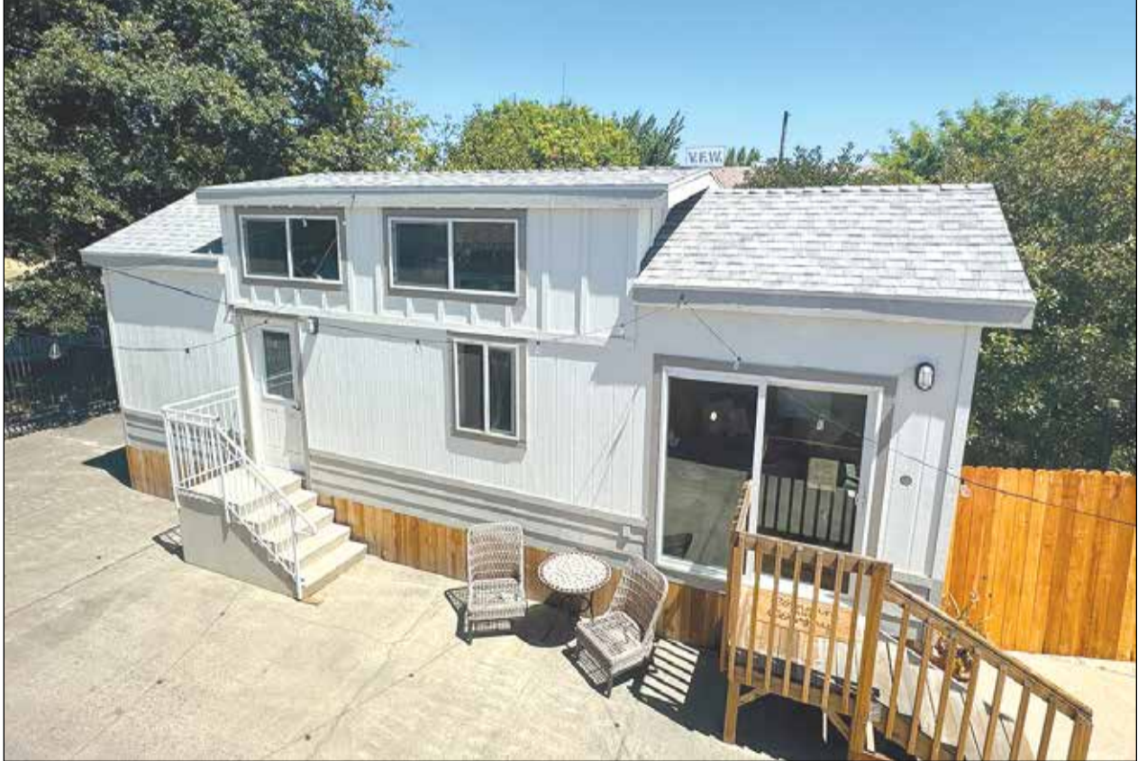
A manufactured home with an upstairs loft is on display at Reliable Home Solutions in West Sacramento.
