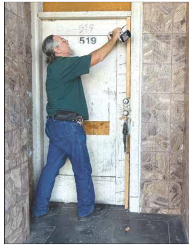
Don Melvin boards up the entrance to an adjacent office building connected to the State Theater in an effort to deter further break-ins. He believes the structure could be converted into several small apartments with the right investment.
