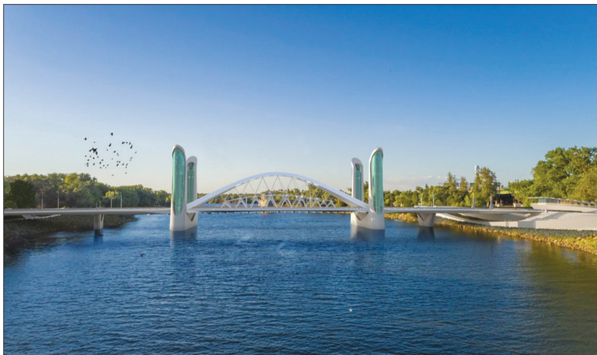
The long-anticipated I Street Bridge Replacement Project is expected to take four years to finish. Construction is expected to begin in spring 2026. Photo courtesy of City of Sacramento
