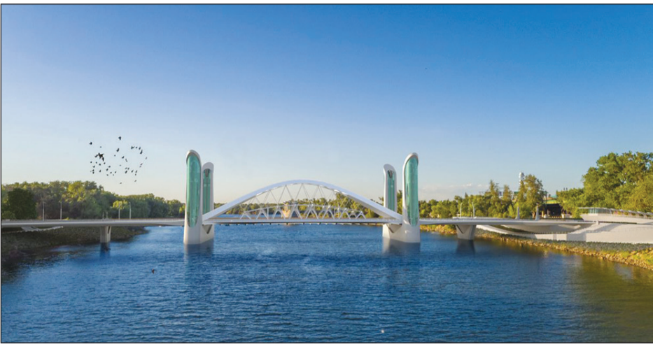
The long-anticipated I Street Bridge Replacement Project is expected to take four years to finish. Construction is expected to begin in spring 2026. Photo courtesy of City of Sacramento
