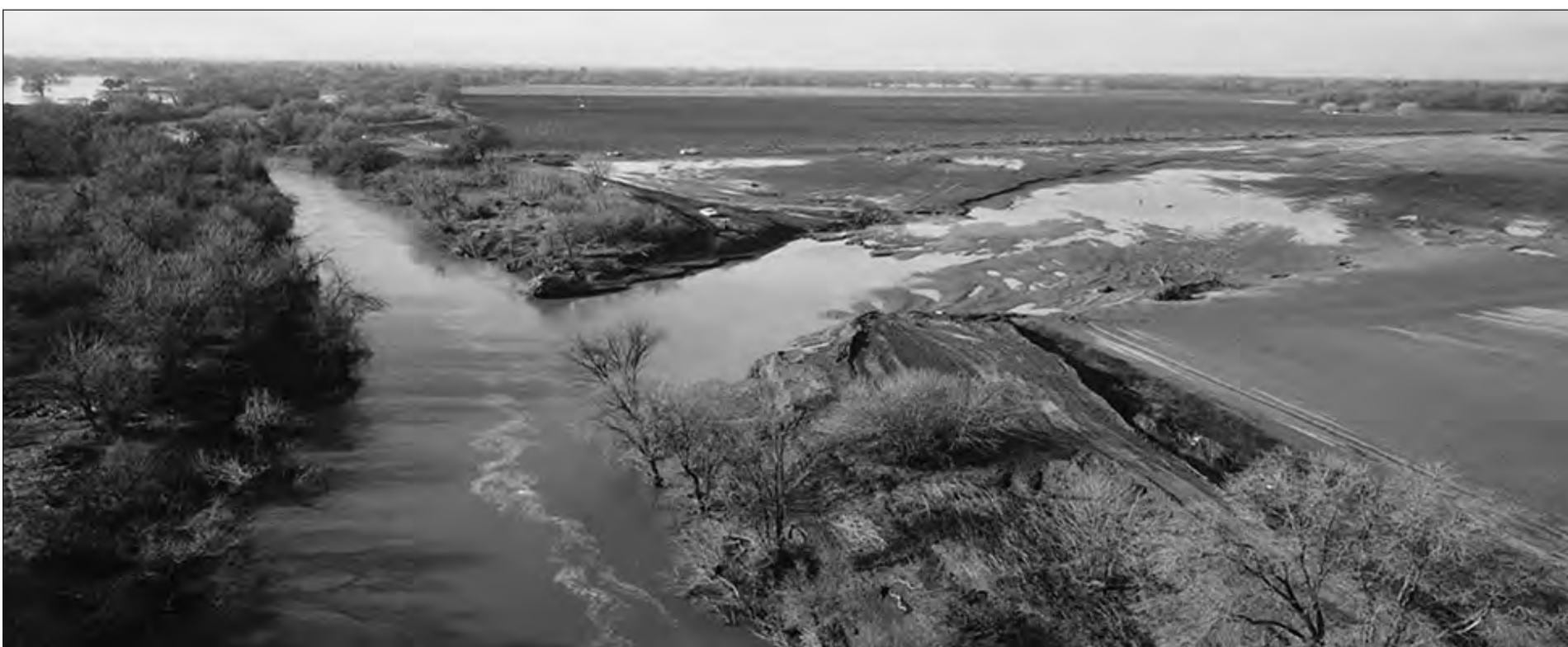
A photo taken after the 2023 flooding shows the most severe of three levee breaks. Located at the end of Bradley Ranch Road in the Sheldon community, the break stretched the length of a football field. Courtesy photo
