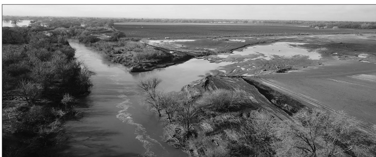
A photo taken after the 2023 flooding shows the most severe of three levee breaks. Located at the end of Bradley Ranch Road in the Sheldon community, the break stretched the length of a football field. Courtesy photo
