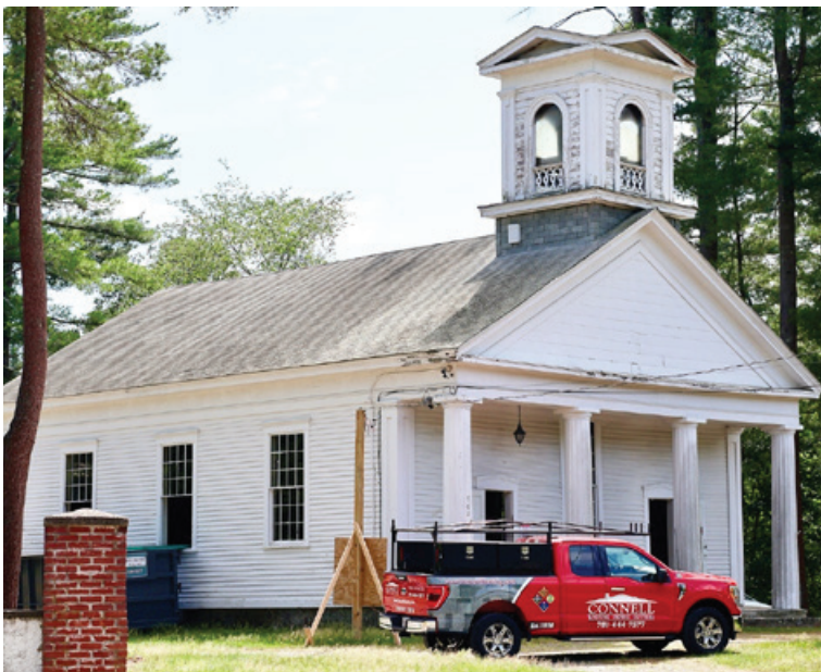
This 1856 building will be converted to needed housing thanks to Franklin CPA funds, Habitat for Humanity and donations from local businesses, such as Connell Roofing.
