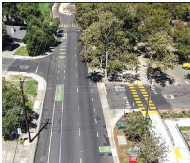
Other major additions to Rancho Cordova's trails system are on the horizon for the City of Rancho Cordova. The Zinfandel Pedestrian Overcrossing is also being designed and construction is anticipated to begin next year. Photo courtesy of the City of Rancho Cordova
