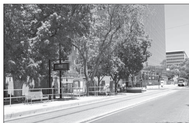
Due to the construction fencing and site limitations, SacRT was unable to raise the east platform during the last phase of light rail station platform upgrades. Photo courtesy of Sacramento Regional Transit District
