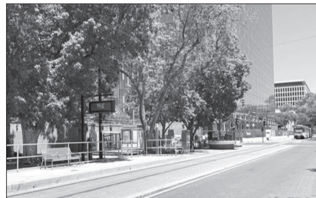
Due to the construction fencing and site limitations, SacRT was unable to raise the east platform during the last phase of light rail station platform upgrades. Photo courtesy of Sacramento Regional Transit District
