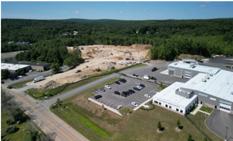
An arial view of the new field construction. Courtesy of Holden Community Television
