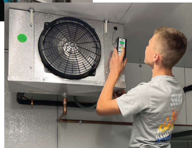
Lincoln Shaw of Northbridge, a junior in the Heating, Ventilation, Air Conditioning & Refrigeration (HVAC&R) program at BVT, helped install the new system.
