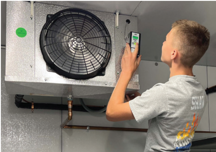
Lincoln Shaw: Lincoln Shaw of Northbridge, a junior in the Heating, Ventilation, Air Conditioning & Refrigeration (HVAC&R) program at BVT, helped install the new system.
