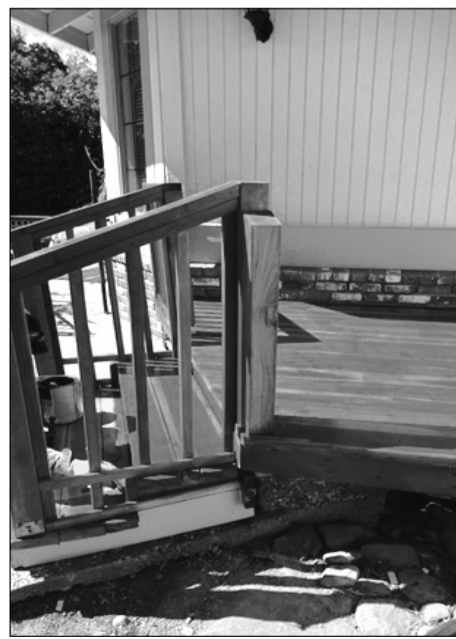
Thanks to the Sacramento County Age-Friendly Community Initiative micro-grant program, repairs such as those to make this deck safe and functional for a Sacramento senior resident were completed. Photo courtesy of Sacramento County
