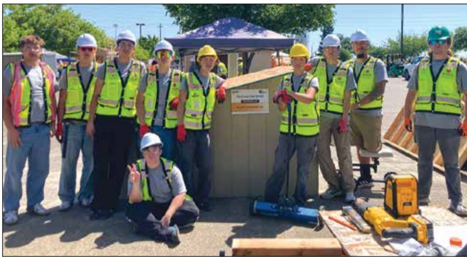
Del Campo High School students faced summer heat, heavy materials and the pressure of working under professional timelines during the 40th annual Design Build Competition. Photo courtesy of San Juan Unified District
