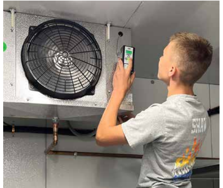
Lincoln Shaw of Northbridge, a junior in the Heating, Ventilation, Air Conditioning & Refrigeration (HVAC&R) program at BVT, helped install the new system. Courtesy photo
