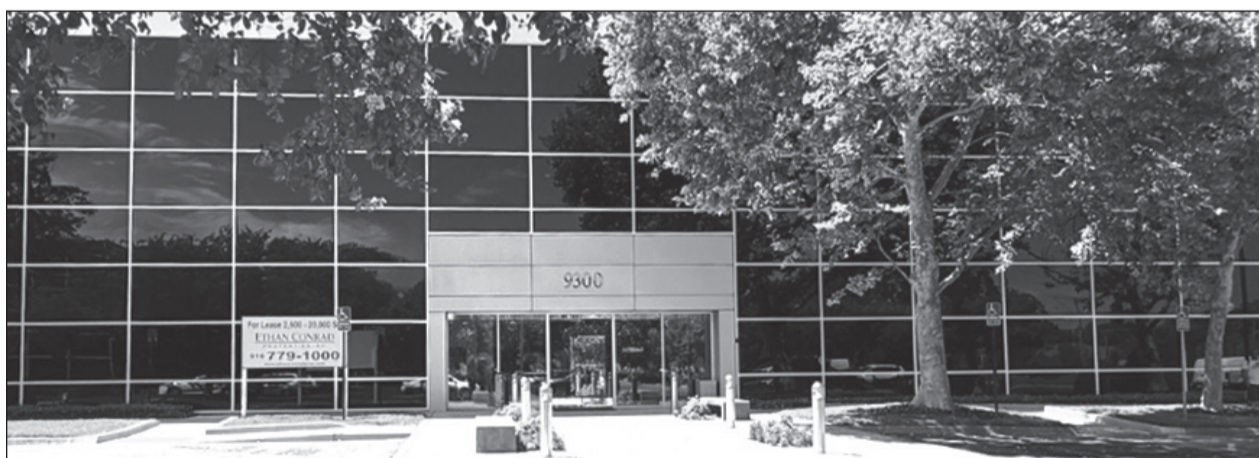
A new exterior drop box is available so that members of the public can turn in their forms after hours. There are currently signs at both the former (3700 Branch Center Road) and new (9300 Tech Center Drive, Suite 100) location to assist the public with the transition. Photo courtesy of Sacramento County
