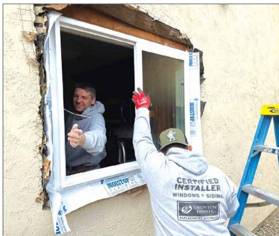
Factory-trained installers "dry fit" a new construction sliding window on a stucco home. One veteran will be awarded a free whole-home upgrade of new Simonton windows and patio doors. Courtesy of California Energy Consultant Service and Simonton Windows.
