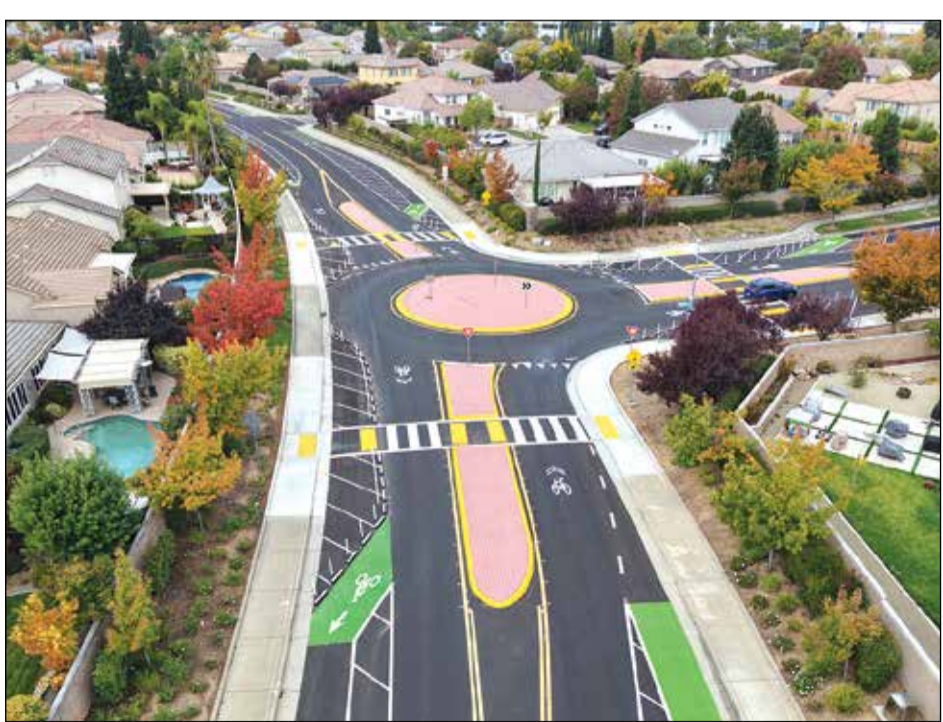
The traffic calming project in the Stone Creek neighborhood on Baroque Drive is intended to reduce speeds and enhance safety along the corridor for motorists, cyclists and pedestrians. Photo courtesy of the City of Rancho Cordova
