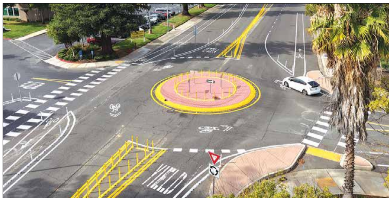
Completed in October, the traffic calming project on Lincoln Village Drive was a result of requests from the community for improvements to enhance safety and reduce travel speeds. Photo courtesy of the City of Rancho Cordova
