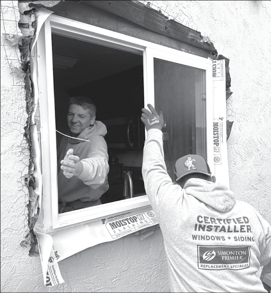
Factory-trained installers “dry fit” a new construction sliding window on a stucco home. One veteran will be awarded a free whole-home upgrade of new Simonton windows and patio doors, courtesy of California Energy Consultant Service and Simonton Windows. Photo courtesy of California Energy Consultant Service
