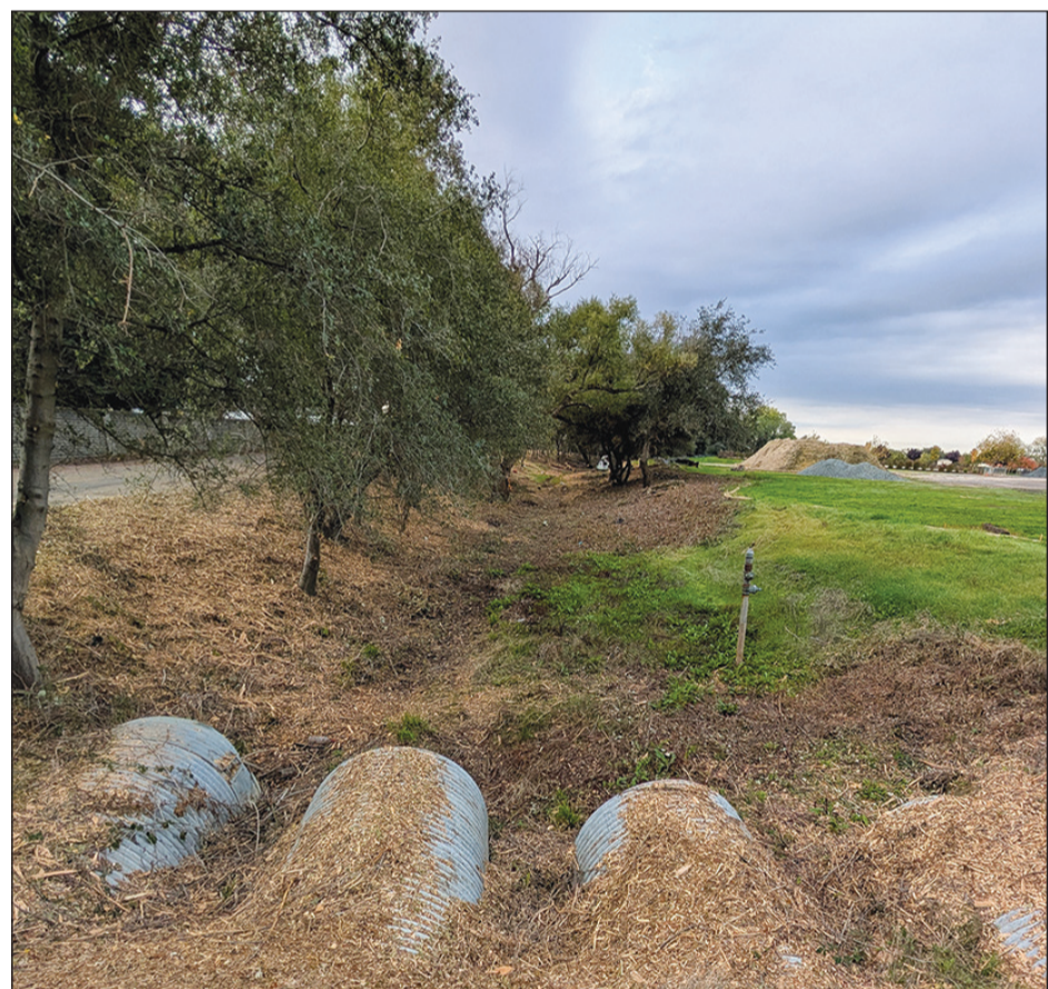
This image shows the ditch after the work.
