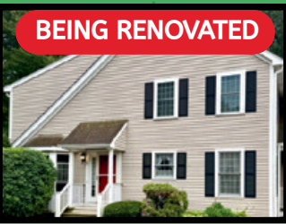
21 Bellwood Cir, Bellingham Being Renovated
