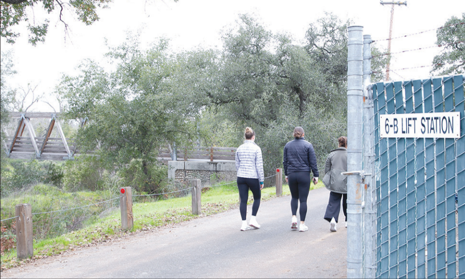
Located near the wooden bridge, Lift Station 6B is operating normally after an emergency in mid-November when the pump couldn't keep up with heavy rain. Photo by Gail Bullen
