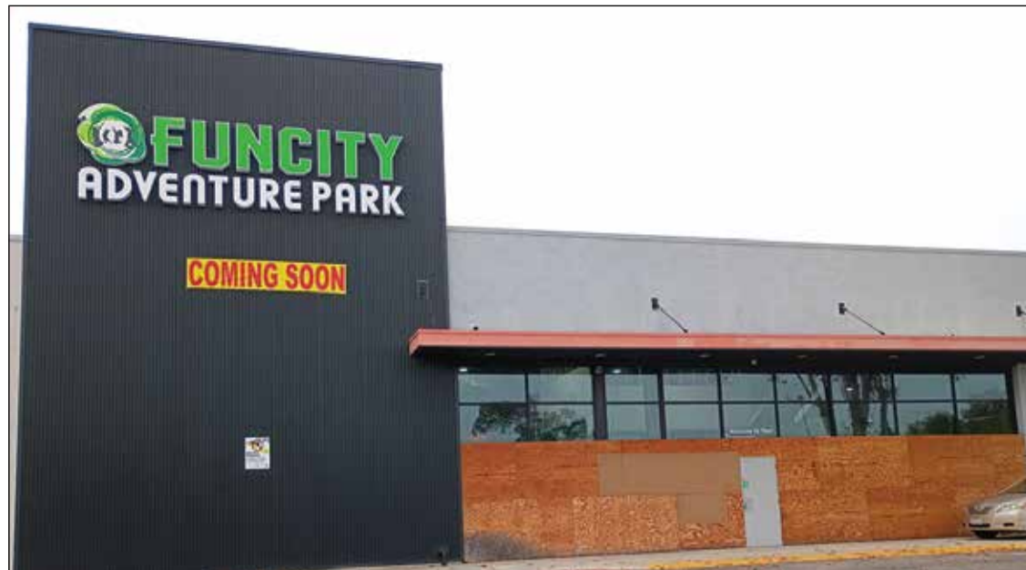
Construction of a new indoor trampoline park, the Fun City Adventure Park at 8525 Auburn Blvd in the Citrus Grove Shopping Center on Auburn Boulevard is nearing completion
