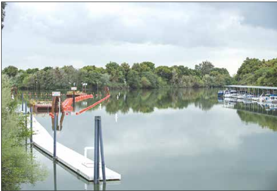
The metal fish barrier for the Georgiana Slough in the activated position on March 27, 2014, in Walnut Grove, CA. Photo courtesy of California Department of Water Resources
