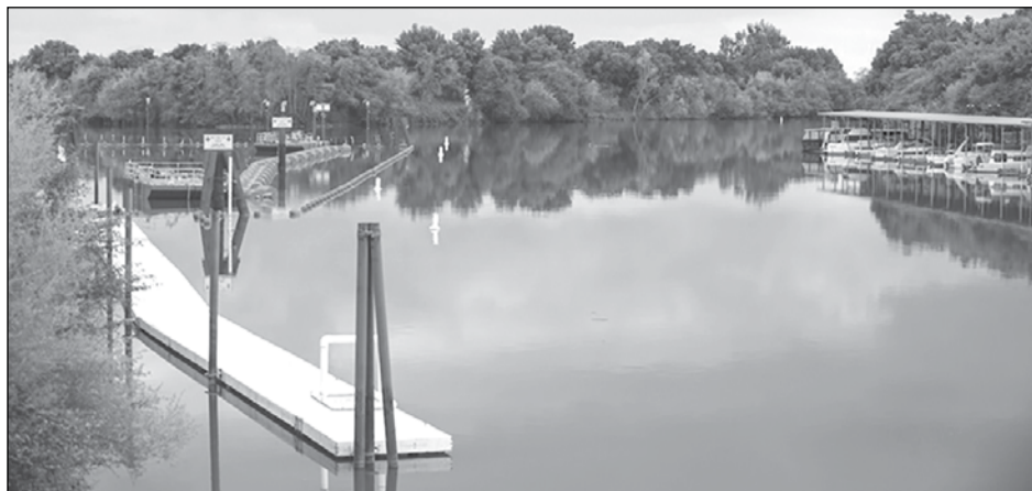
The metal fish barrier for the Georgiana Slough in the activated position on March 27, 2014, in Walnut Grove, CA. Photo courtesy of California Department of Water Resources
