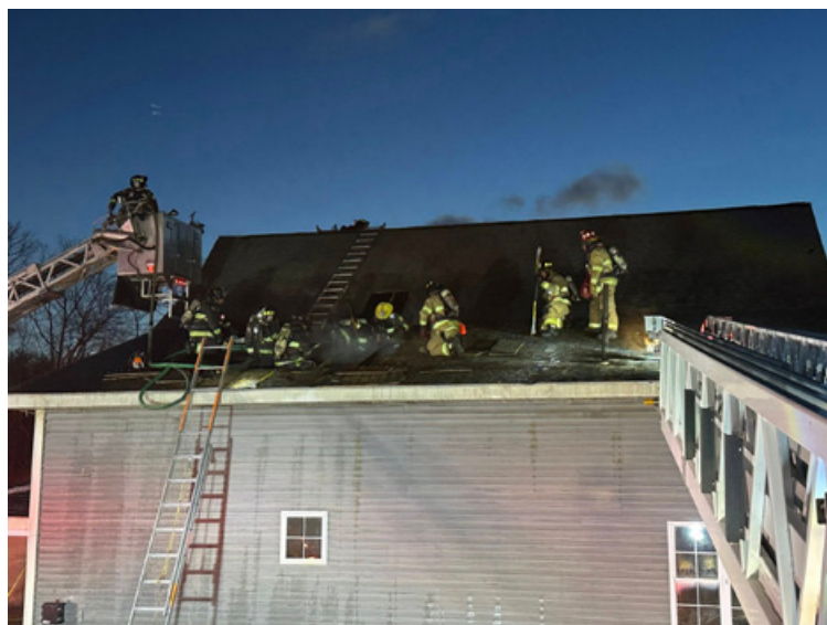
An effort is ongoing to support the business. Photo courtesy Sterling Fire Department.
