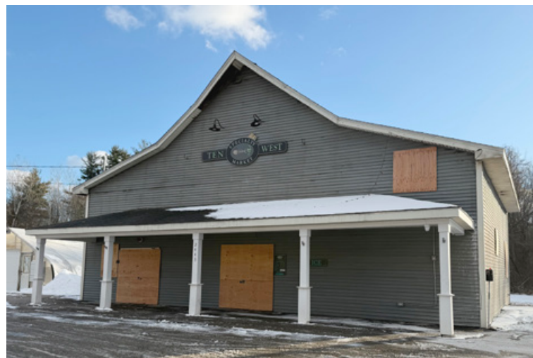
Ten West Market is boarded up following the Dec. 30 fire.
