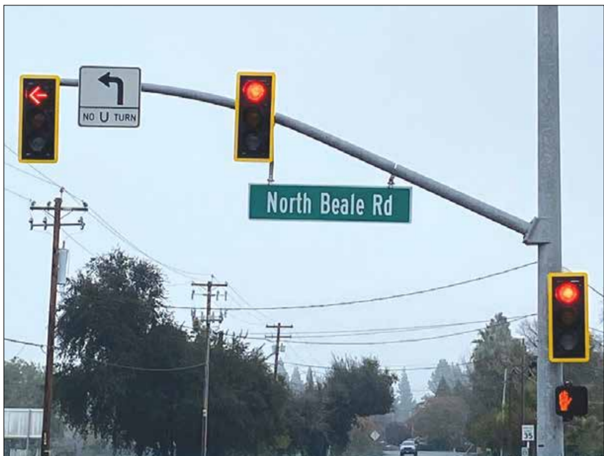
Nine intersections are about to get safer with the Signal Systems Upgrade Project. Photo courtesy of Yuba County
