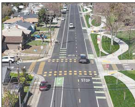
Pictured is the Chase Drive and American River Parkway Connection project which added a multiuse path along the east side of Chase Drive from Coloma Road to the American River Parkway. Photo courtesy of the City of Rancho Cordova
