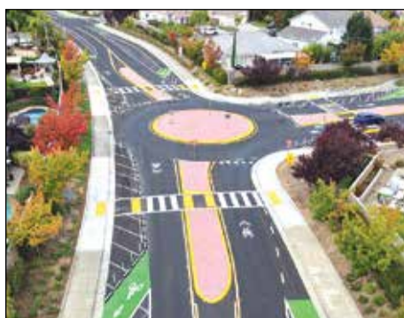
The Baroque Traffic Calming project improvements in the Stone Creek neighborhood on Baroque Drive included a mini roundabout, improved crosswalks, new bike lanes, lane narrowing and surface treatments to enhance safety for motorists, cyclists and pedestrians. Photo courtesy of the City of Rancho Cordova
