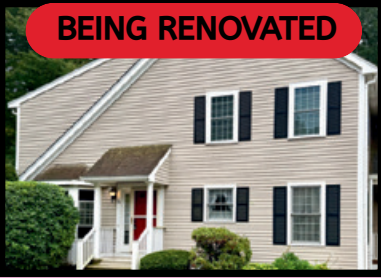
31 Bellwood Cir. Bellingham Being Renovated
