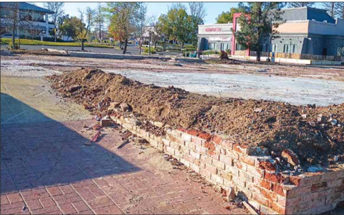
The unevenly cut, thick stumps of multiple young trees which once provided a generous canopy of lush foliage have left the concrete slab on which the restaurant once sat wide open to the blue morning sky.
