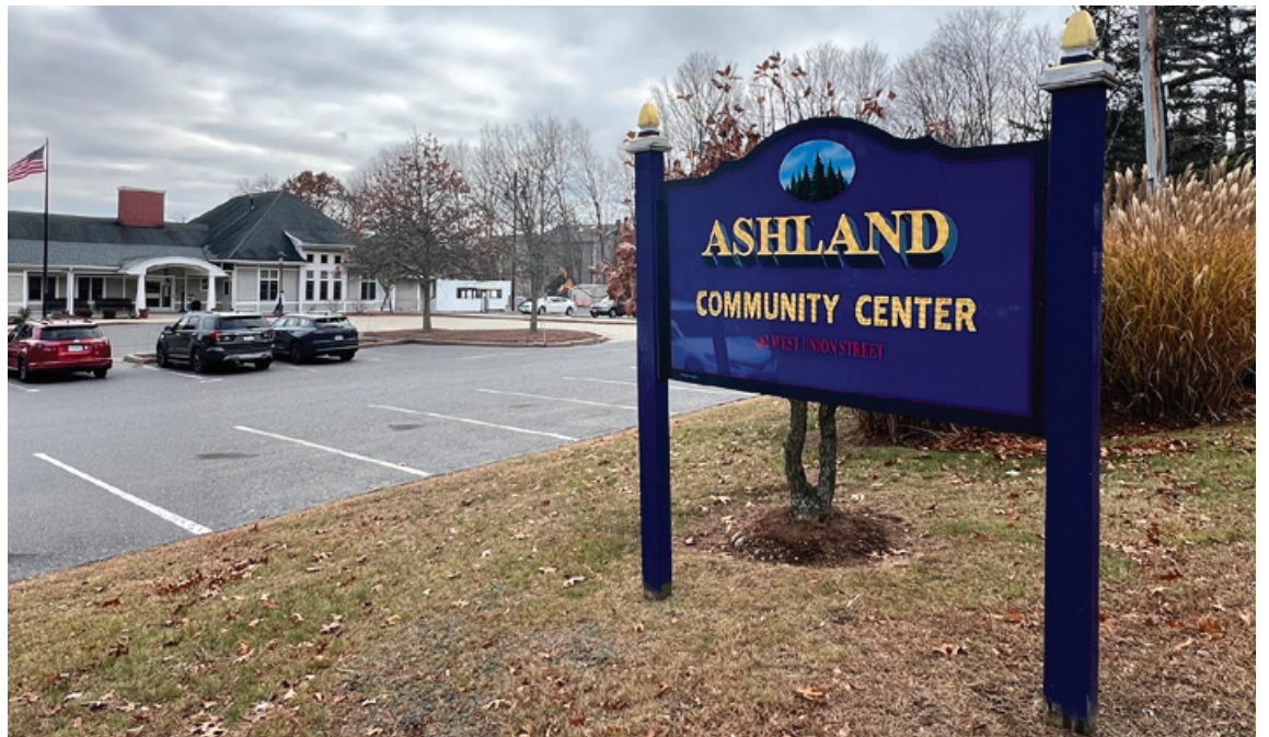
Ashland Community Center which houses the Ashland's Senior Center. Photo by Wendy Watkins
