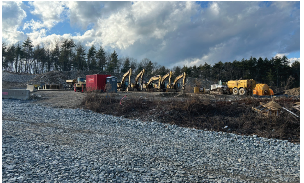
Construction entrance on Pond Street, with grading complete and equipment staged.
