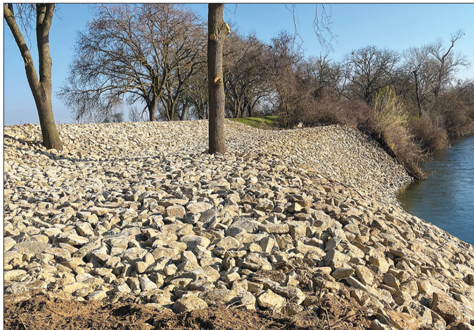
Completed emergency repairs to a levee south of the Folsom South Canal on the Sheldon side of the Cosumnes River are shown after heavy rains in early January. Courtesy photo
