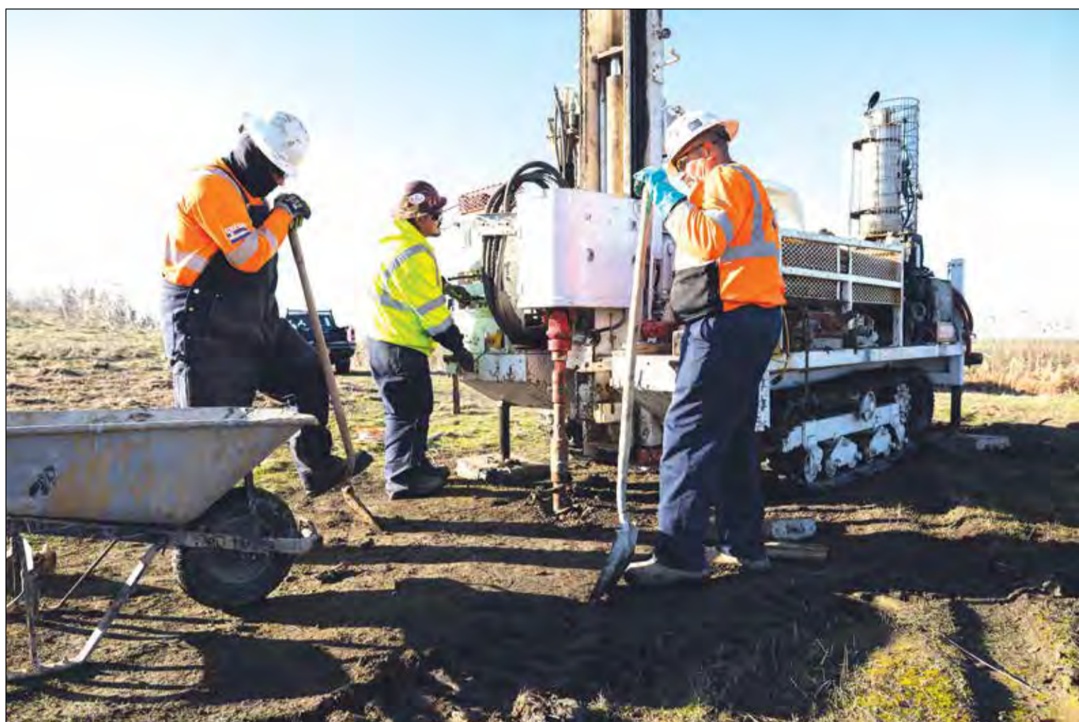
California Department of Water Resources’s Sustainable Groundwater Management Office installs new equipment to enhance the monitoring and understanding of land subsidence in California. The newly installed GPS station and remote sensing calibration equipment will be firmly anchored into the ground to ensure precise positioning and detect vertical movement of the Earth’s surface. Photo by Andrew Nixon / Department of Water Resources
