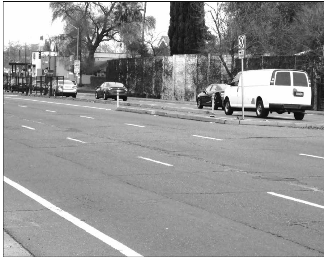
Portions of the fencing barrier along Greenback Lane towards Birdcage Lane destroyed in prior traffic accidents have been gone for at least three years.
