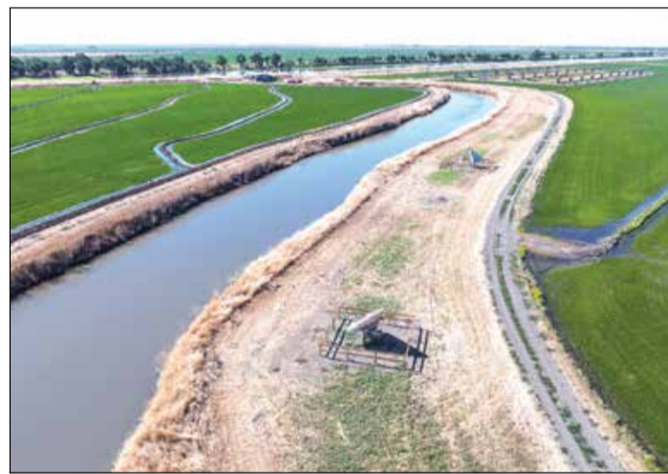
A drone view of newly installed equipment from the California Department of Water Resources' Sustainable Groundwater Management Office to enhance the monitoring and understanding of land subsidence in California. The newly installed GPS station and remote sensing calibration equipment are firmly anchored into the ground to ensure precise positioning and detect vertical movement of the Earth's surface. Photo by Nick Shockley / California Department of Water Resources
