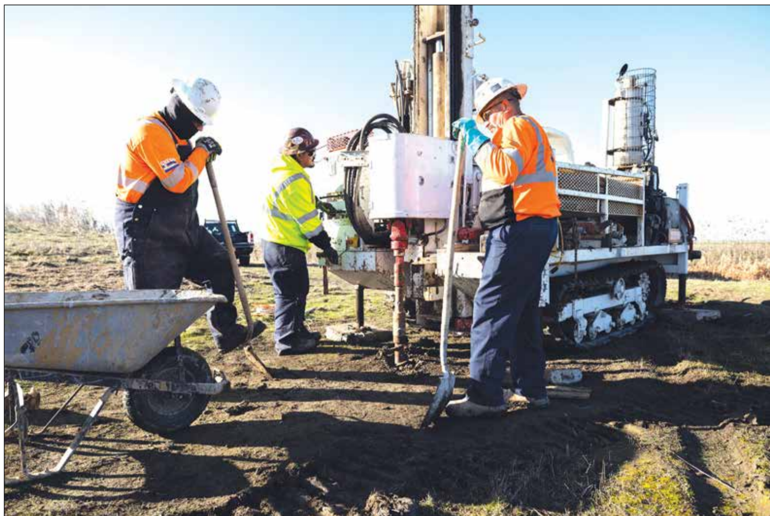
California Department of Water Resources's Sustainable Groundwater Management Office installs new equipment to enhance the monitoring and understanding of land subsidence in California. The newly installed GPS station and remote sensing calibration equipment will be firmly anchored into the ground to ensure precise positioning and detect vertical movement of the Earth's surface. Photo by Andrew Nixon / Department of Water Resources
