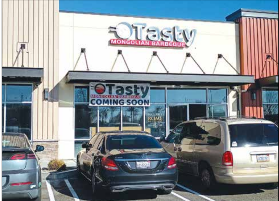
O Tasty Mongolian BBQ, now under construction in the Copperwood Square Shopping Center in Citrus Heights is looking to open in March. Photo by Thomas J. Sullivan
