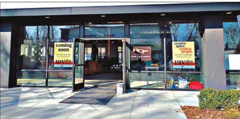
My Salon Suite, now under construction, will fill a 7,334-square-foot retail building next to Sierra Laundry at 7811 Madison Avenue in the Sunrise Village Shopping Center at the northwest corner of Madison Avenue and Sunrise Boulevard.
